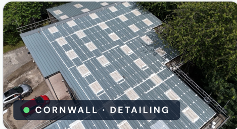
Fig 4. Asbestos cement at Clarkes 24/7, Bristol (silicone only) and profiled metal at Tresidder Close, Cornwall.
