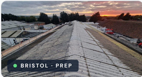
Fig 4. Asbestos cement at Clarkes 24/7, Bristol (silicone only) and profiled metal at Tresidder Close, Cornwall.
