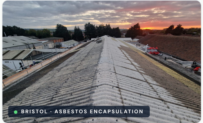
Fig 2. Prep under way on the Clarke's 24/7 asbestos roof, Bristol — biocidal clean and detailing from crawl boards, sheets never cut, drilled or abraded.
