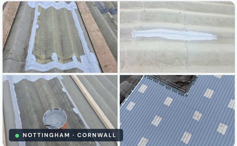
Fig 3. SF42 seam-sealing in the field — a rooflight perimeter and laps sealed on corrugated cement fibre at Nottingham (worked from crawl boards), and every lap, fixing and rooflight sealed at Tresidder Close, Cornwall.
