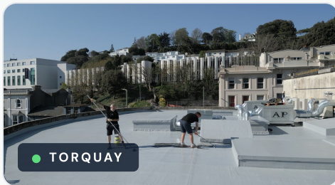
Fig 4. Recent UK installations of the GacoFlex S42 system on the South Coast — seamless, monolithic, single-coat silicone membrane covering existing flat roofs.
